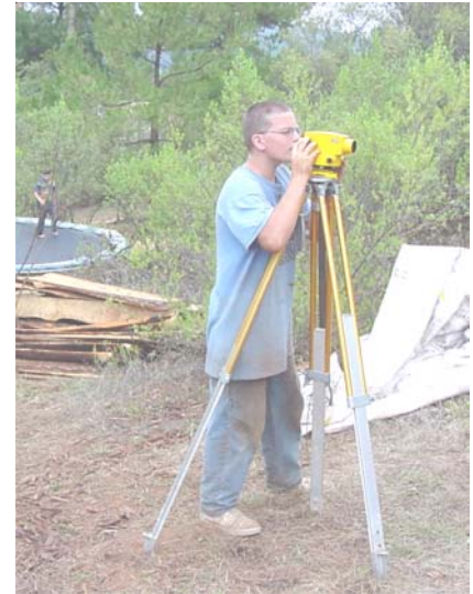
Caleb at the level, shooting the foundation for the first dome.
