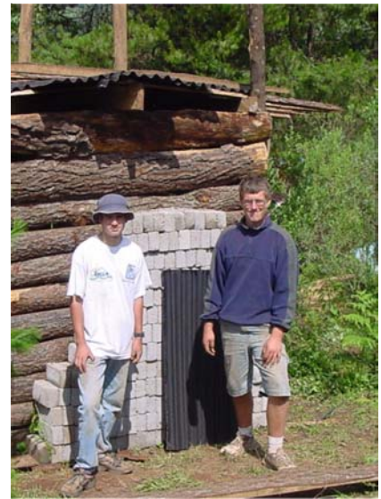
Marlon & Nathan in front of their creation--a rustic storage shed for camp construction equipment.
